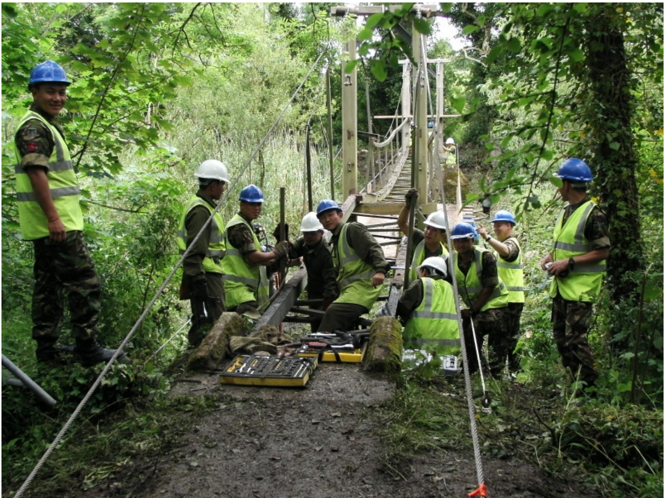
Dismantling the North Stoke suspension footbridge May 2009
